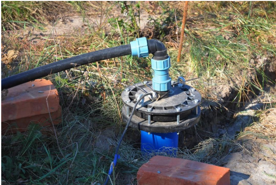
Figure 4.12: Shallow Bore Typical Arrangement
